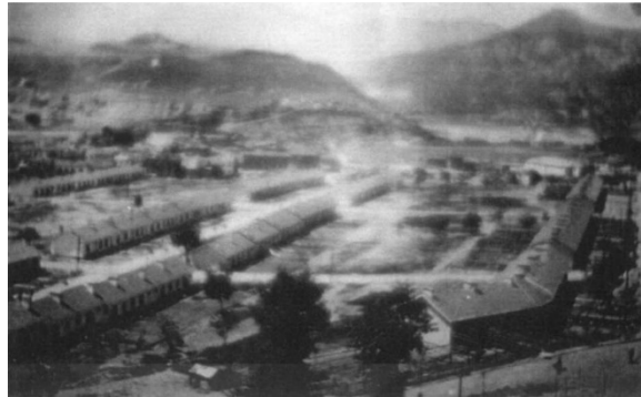
Figure 15: Karabük Iron and Steel Works Settlement, workers' row houses, undated (Öktem, 2004, 98).
