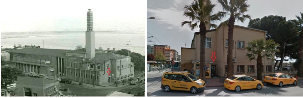
Figure 15 (Left): Izmit People's House frontal view and the library entrance (URL-4).
