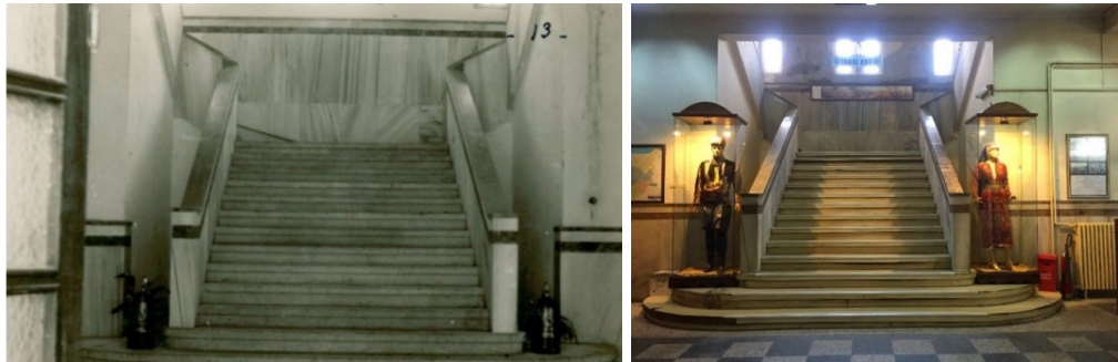
Figure 17 (Left): Izmit People's House ground floor stairs view (IHEM Archive, URL-6).
