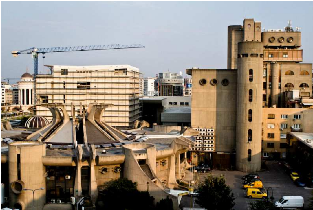
Fig. 10: The Central Post Office, designed by Janko Konstantinov (URL-5)
