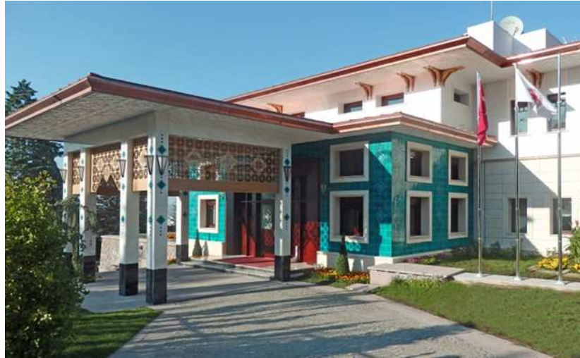
Figure 23: TGNA Prime Ministry official Residence (URL-18).
